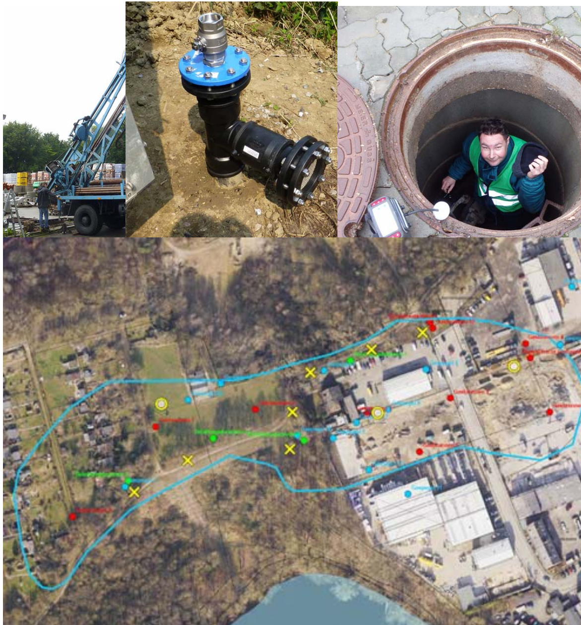
Illustration 6: TOP: Machine systems of the abandoned "Kiel – Drachensee" waste disposal site (on the left) and the implementation of drilling operations in the industrial area of the abandoned waste disposal site (in the middle) and on the right: new aeration well At the BOTTOM: Overview of the measures at the abandoned waste disposal site with aeration wells, gas wells and gas levels.
